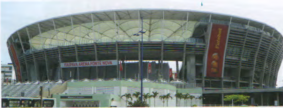
This outside view of Arena Fonte Nova, in Salvador, Brazil, shows the high-walled construction typical of stadiums with high seating capacities and a prime factor in the shade issue.
